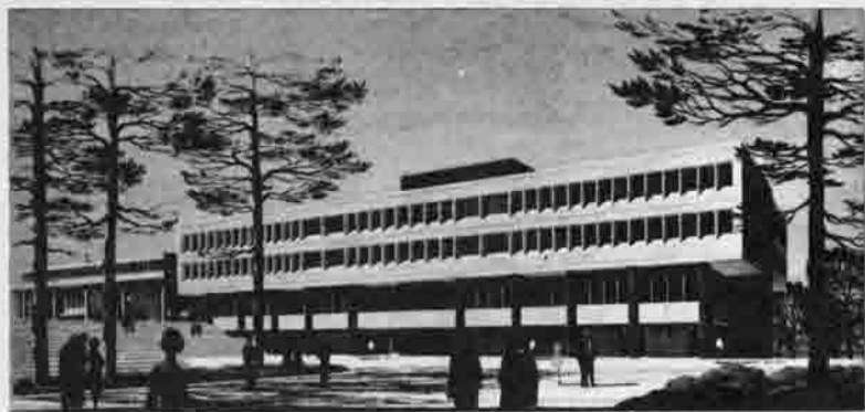
The architect's concept of the Arts and Science Building for $1 million is shown above. The Math-Language Building is in the background at the right.
